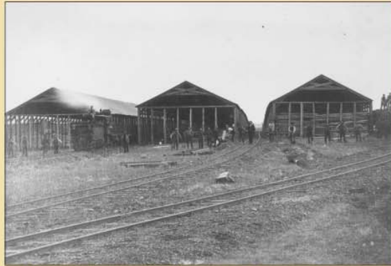
Coal deteriorated rapidly when exposed to the air. Sheds such as these at Dunmore, near Medicine Hat were erected to protect the coal from the elements. Sir Alexander Galt Museum & Archives
