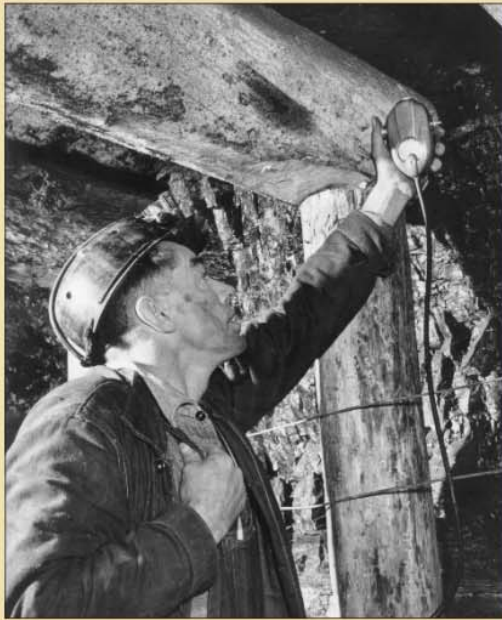
Tests were made for methane gas prior to workmen entering an area. This is a posed photo, as the test must have already been made. An exploding flash bulb could have caused an explosion if gas was present.
