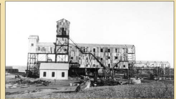
Head frame of Galt No. 8 Mine, 1935
