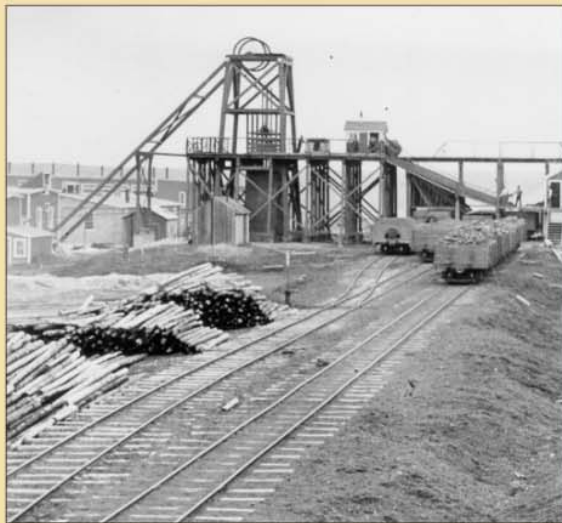
Galt Shaft #1, showing cars being loaded with lump, nut and slack coal. Alberta Railway & Coal Co. Lethbridge, N.W.T.
