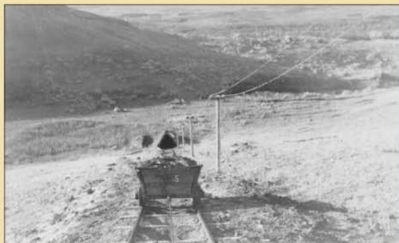
An inclined railway such as this one was used to bring the coal out of the river valley from the Lethbridge Coal Co. mine.
