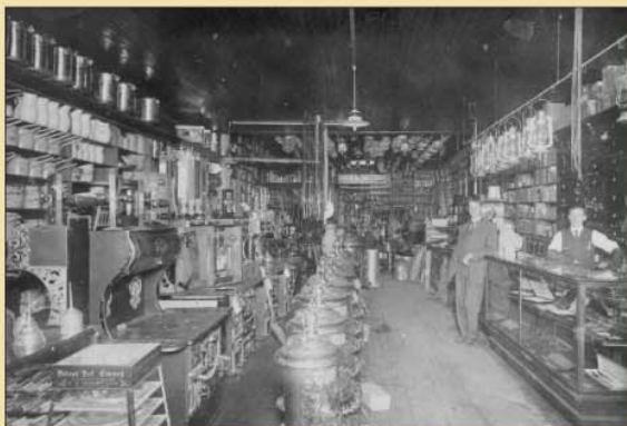
Interior of J.M. Taylor's hardware store showing a selection of coal kitchen ranges and coal heaters used during the coal era.
